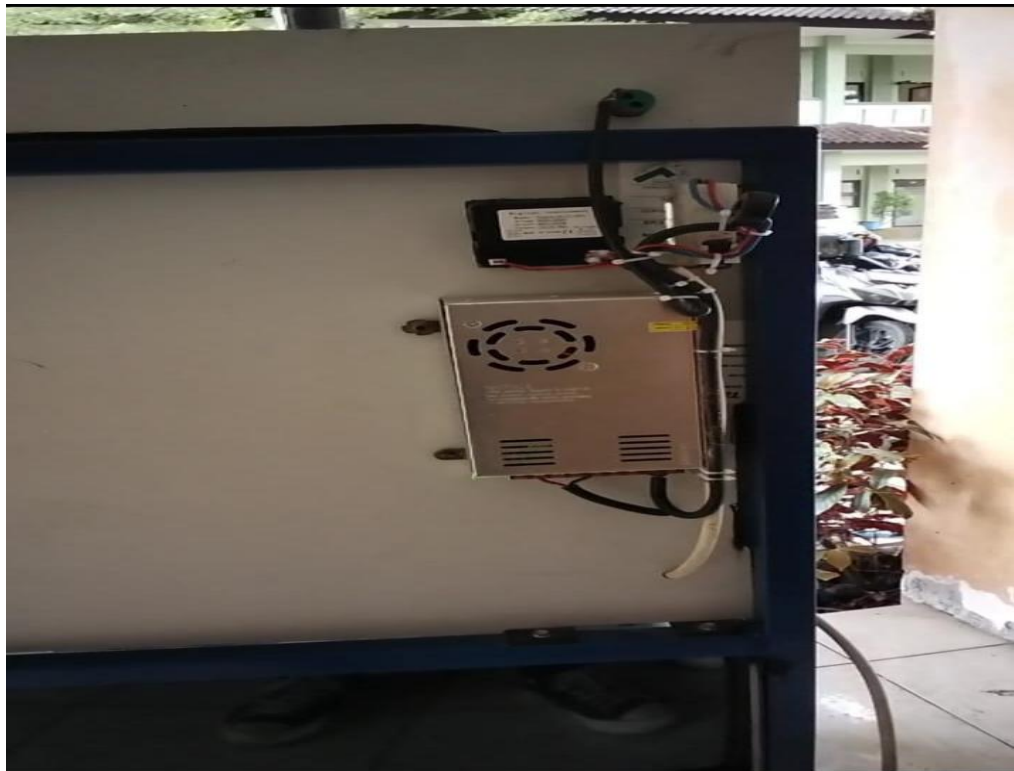
Lampiran 7 Pemasangan power supply
